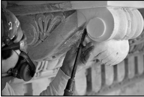
Figure 7. Marble dutchman patches were carved in place
