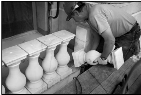
Figure 8. New turned marble balusters were installed at all balconies and parapets
