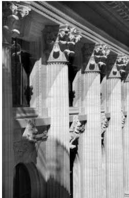
Figure 9. Detail of completed front facade
