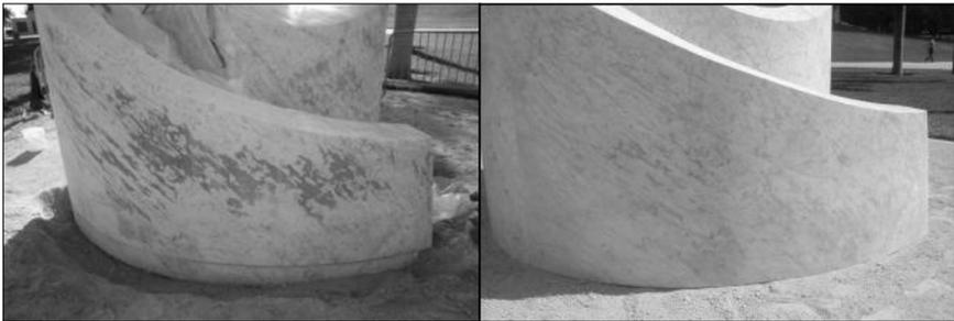
**Figure 1, 2.** Disfiguring biological staining before (left) and after (right) treatment with CB-4 bacteriostatic detergent.
