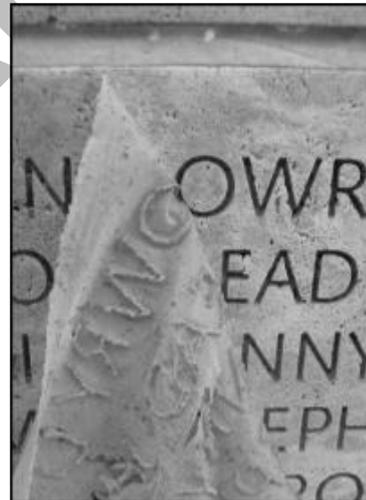
**Figure 3.** Prestor gel being pulled from the surface of the National Law Enforcement Officers Memorial, Washington, DC.
