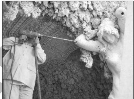
**Figure 6 (above).** Core drilling a sculpture to facilitate installation of a grouted anchor.
