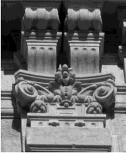
**Figure 2.1.** Example of sculpture made of natural cements and located on the fronts of a residential building.
