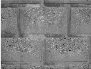
**Figure 2.4.** Example of erosion phenomenon on a cast concrete block from a wall in Grenoble.
