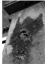
**Figure 2.5.** Spalling phenomenon associated with black crust on the Champollion high school in Grenoble.
