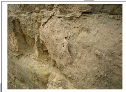
**Figure 6.** Large scaling due to salt crystallization near the stone surface.
