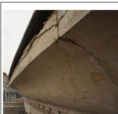
**Figure 4.** Large crack propagation along a cornice
