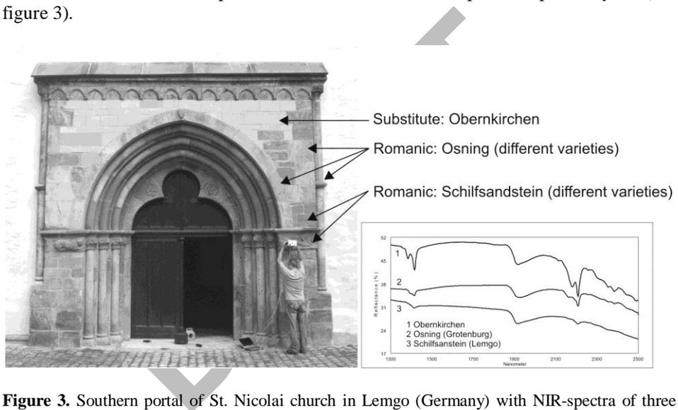
**Figure 3.** Southern portal of St. Nicolai church in Lemgo (Germany) with NIR-spectra of three used building sandstones
