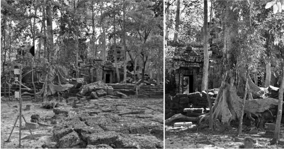
**Figure 2.** The West side of Ta Nei temple, where one of the microclimatic stations was settled. Note the diffuse collapses and cracks on the walls, and stone surfaces widely covered by different biological colonisations.
