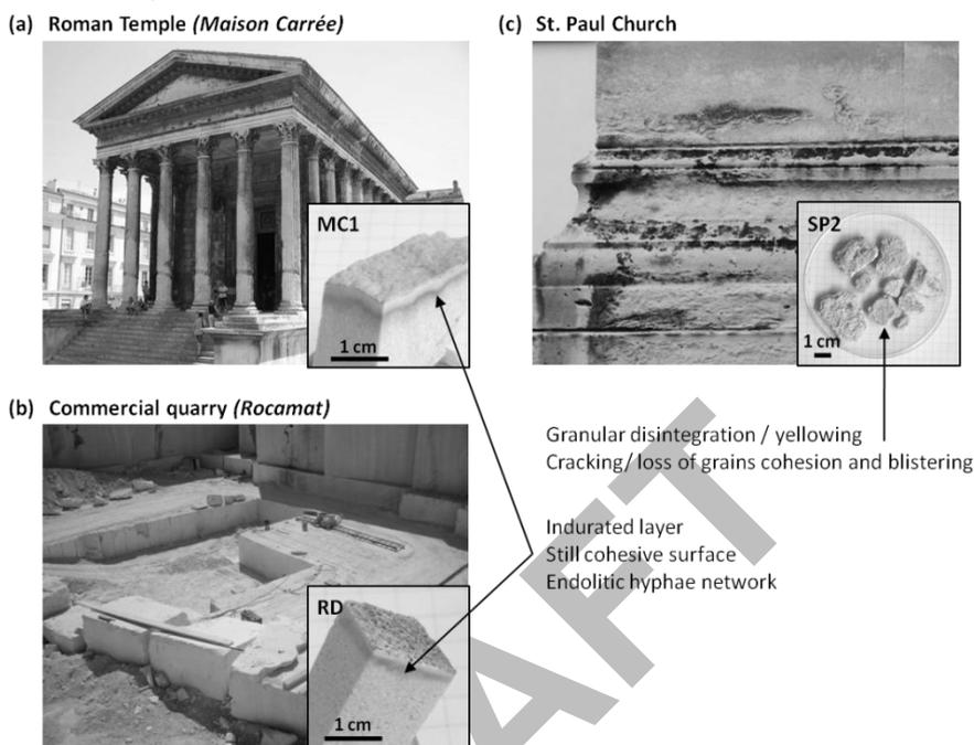
**Figure 5.** Photographs showing three different patinated samples of Bois des Lens stone. (a) The façade of a Roman temple dating from the 1st century after JC in Nîmes downtown (Maison Carrée) and detail of a patinated sample (MC1). (b) Stone quarry currently in operation and details of a sample taken from a 50 years working face (RD). (c) Front of St Paul's Church showing blistering, yellowing and granular disintegration.
