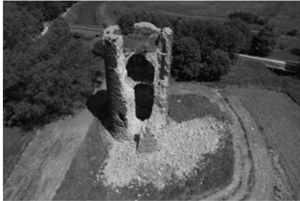
**Figure 2.** Virgin Tower at Zichem, an abandoned medieval four stage dungeon erected in the 14th century, after its partial collapse in 2006 due to loading by roof breakdown, important soil deposit and long-lasting water infiltration. The structure has since been consolidated in its present form and protected against further infiltration. The present study deals with the standing walls not affected by the collapse.
