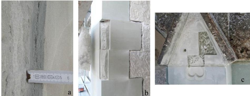
**Fig. 1** (a) Common dimension of spalling in a molasse sandstone - (b) and (c) Application of the artificial stone as a repair material.
