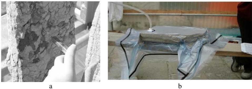
**Figure 1.** Consolidation with fluid inorganic mortars on the thin spires of the roof of the Doge's palace (a) epoxidic treatment in San Geremia Church (b).
