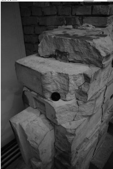
**Figure 3.** Fire damage on masonry, Lepsius Bau, Dresden.
