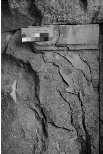
**Figure 1.** Loss of pieces of several cm in thickness parallel to surface, typical fire damage, Dresden, Palais im Großen Garten.
