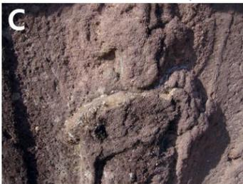
**Figure 1. (C)** Granular disintegration of the basement stone
