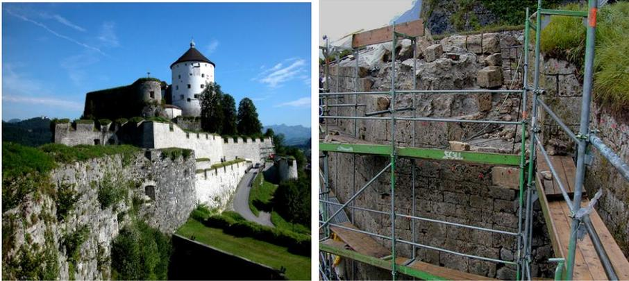
**Figure 2.** The fortress of Kufstein/Tirol (left); the outer fortification walls are constructed from Thiersee tufa. Remedial maintenance of the fortification wall (right).
