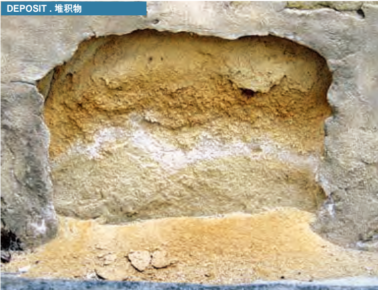
The material detached from the sandstone block forms a deposit . 从砂岩石材上剥落下来的物质形成的堆积物。
