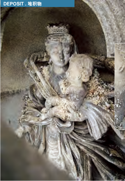
Deposit of pigeon droppings on granite sculpture. 花岗岩雕塑上鸽子粪形成的堆积物。
